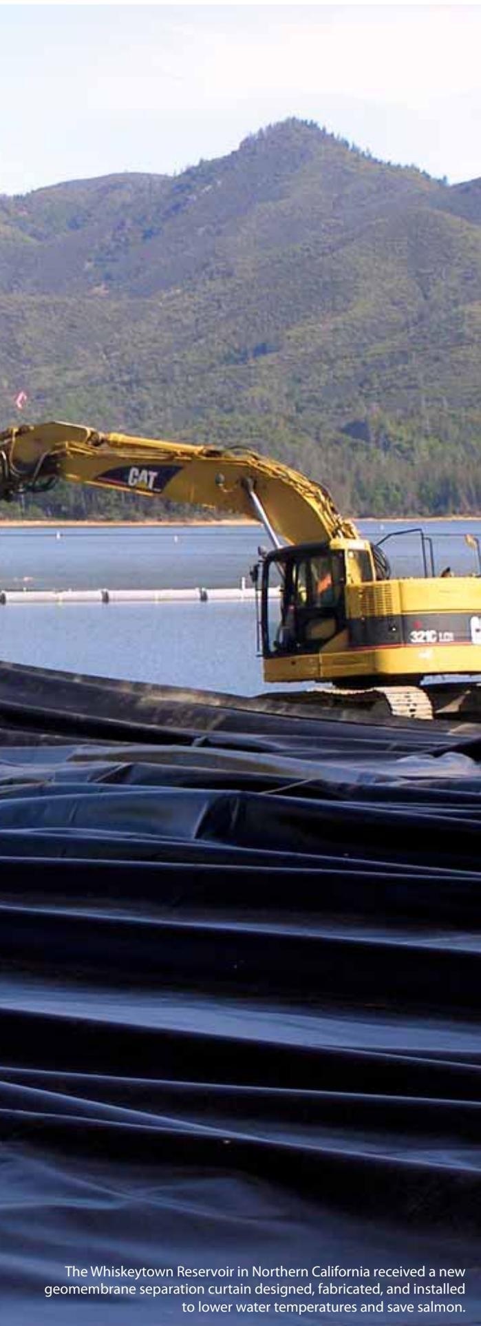
The Whiskeytown Reservoir in Northern California received a new geomembrane separation curtain designed, fabricated, and installed to lower water temperatures and save salmon.
