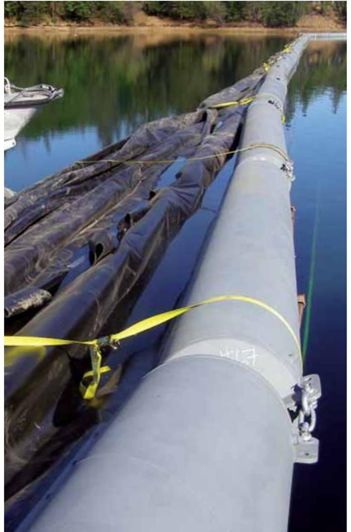
FIGURE 8 Metal floats in place and curtain ready to be anchored to the river bottom by 800-lb weights
