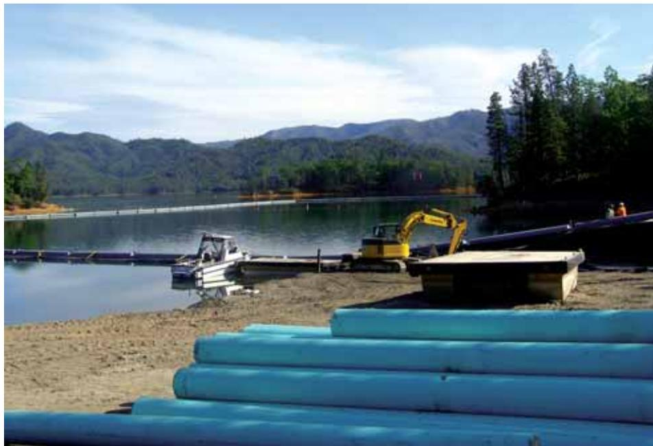
FIGURE 5 800-lb metal weights (foreground) used to secure the curtain
