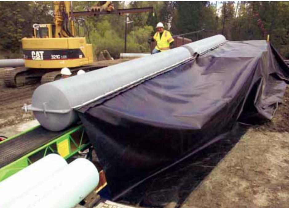
FIGURE 6 Geomembrane curtain was clamped in the metal floats before being deployed
