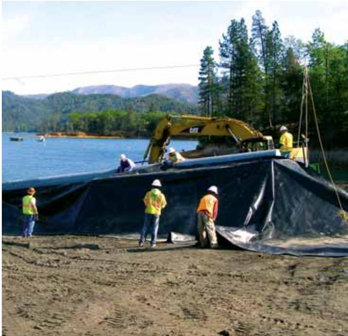
FIGURE 2 Assembly of the curtain on the shoreline
