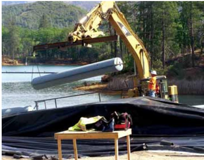
FIGURE 4 Crane setting a float onto the frame
