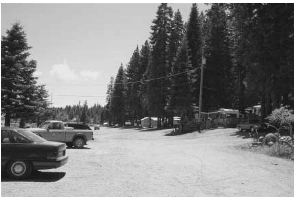
Photo 14. Power line crossing at Plumas Pines boat ramp.
