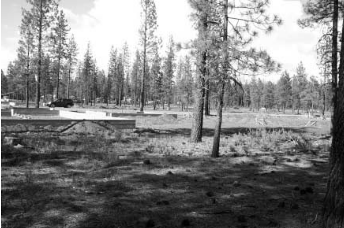
Photo 23. Vision Lake Homes subdivision under construction as of the inspection.
