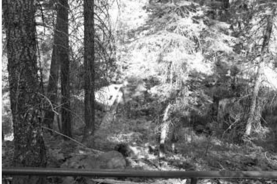
Photo 1. Control weir on North Fork Feather River below Almanor Reservoir at Gage No. NF-2.
