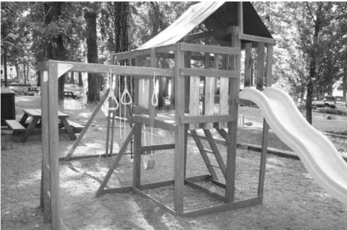
Photo 10. Child play structure at Northshore Campground had loose connections, sharp edges, and exposed bolts. It was removed after the inspection.
