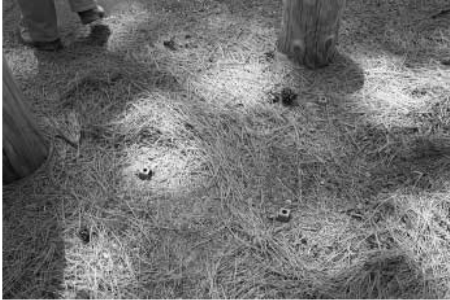
Photo 11. Abandoned trash can anchors represented a tripping hazard.
