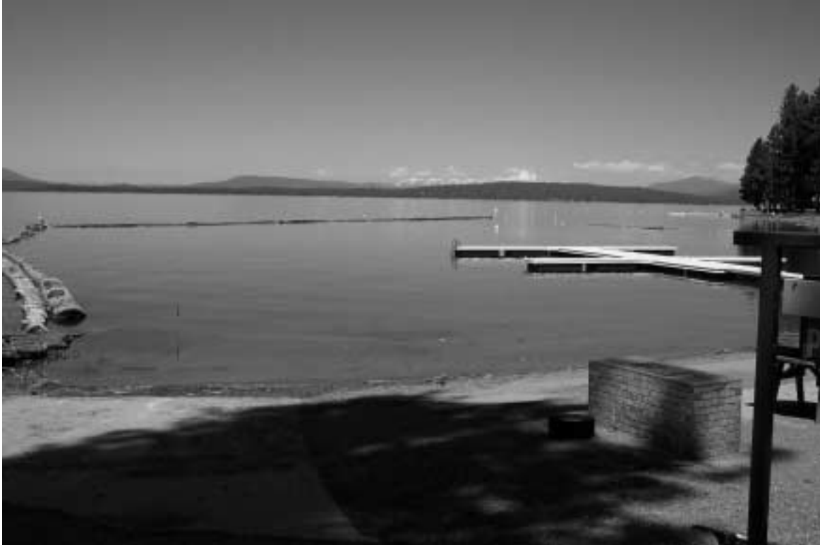
Photo 7. Typical low-visibility partially sunken log booms at Lake Almanor Reservoir.
