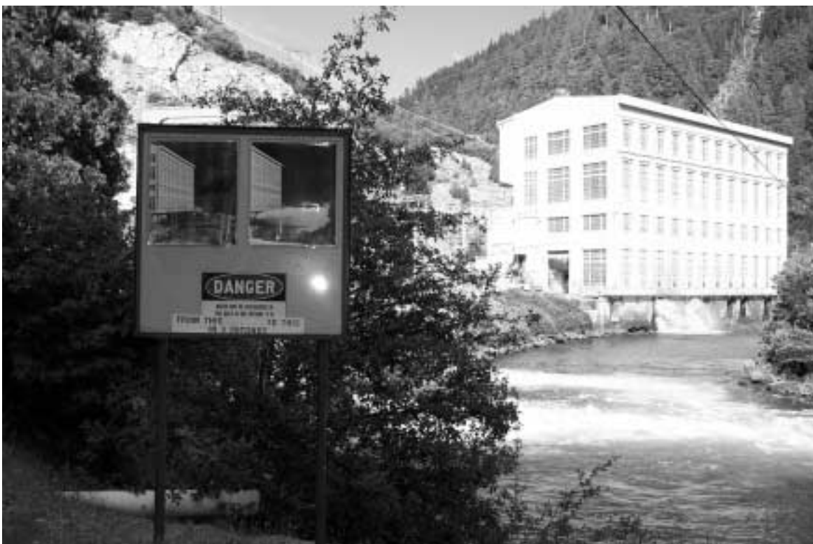
Photo 8. Sudden water fluctuation warning signs at Caribou Powerhouse with large before and after photos.
