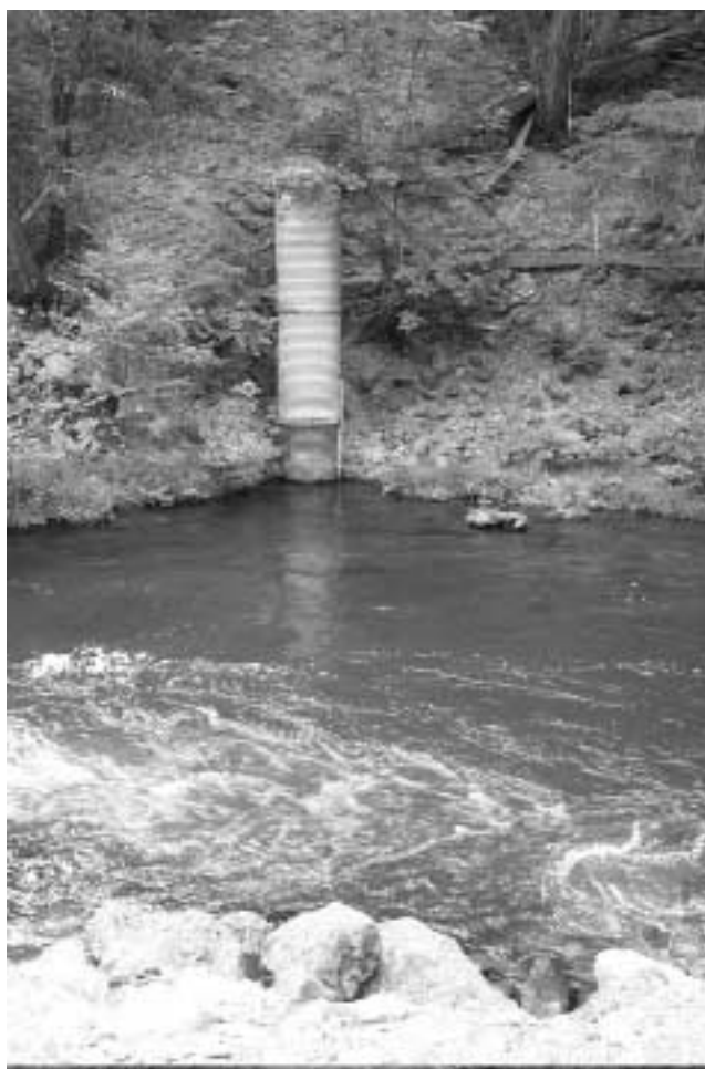
Photo 2. Gaging Station No. NF-70 on North Fork Feather River below Belden Forebay.
