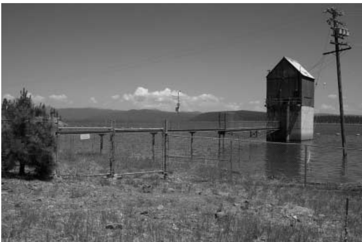
Photo 24. Prattville Intake in Lake Almanor Reservoir. Note public exclusion safety fencing.
