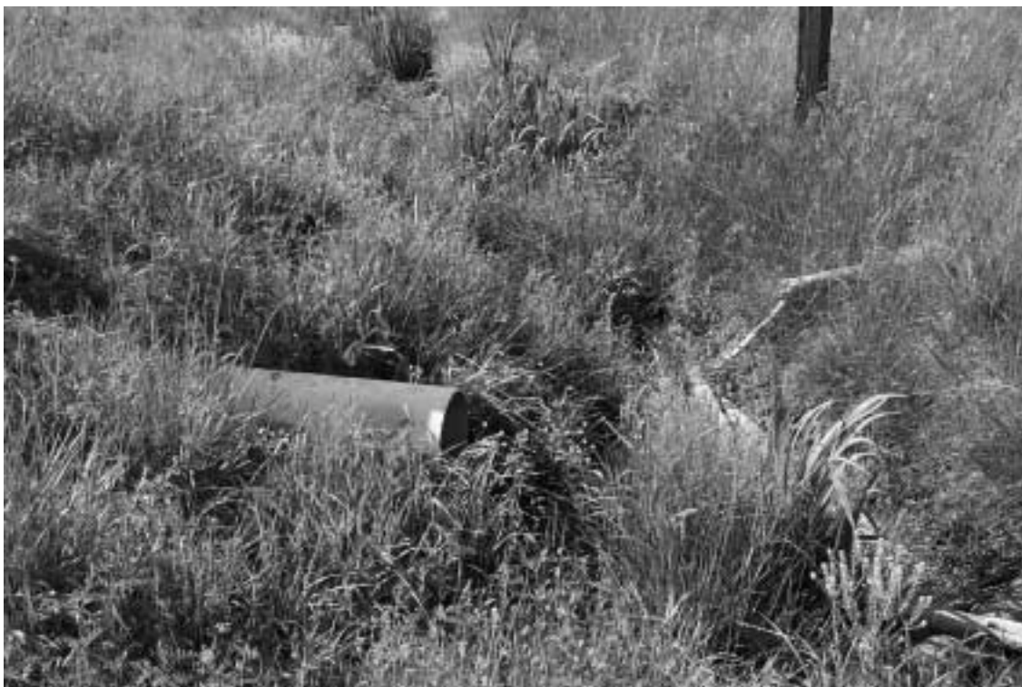
Photo 17. Outfall from wetland pond to drainage ditch that discharges to Lake Almanor Reservoir.
