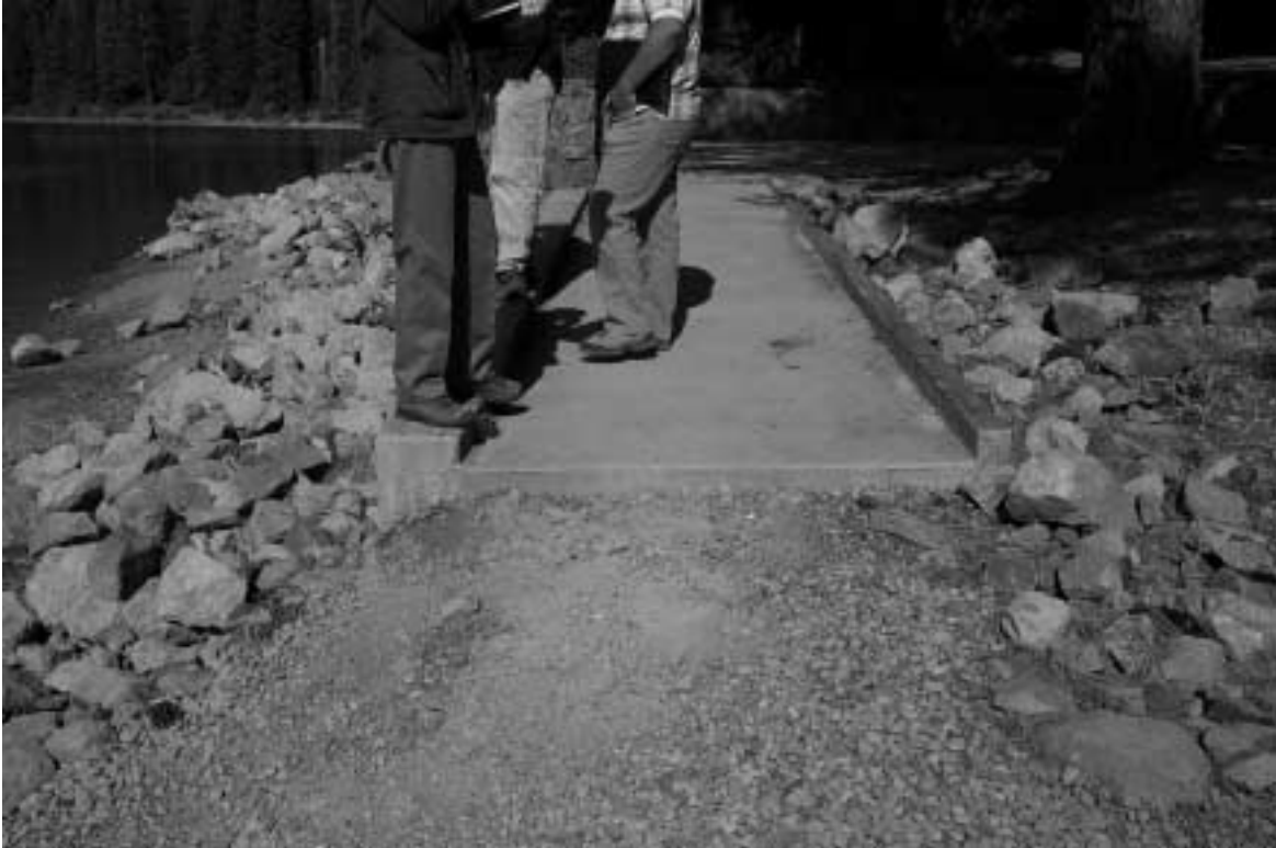
Photo 9. Lip and gravel at end of new accessible ramp at the Canyon Dam picnic area.
