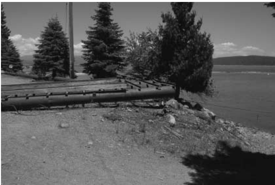
Photo 18. Debris at Plumas Pines Resort was removed after the inspection.
