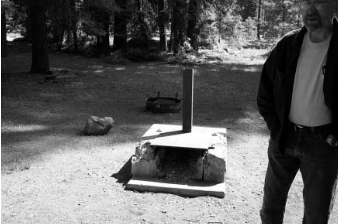
Photo 21. Deteriorated Klamath stoves will be replaced by the next recreation season.
