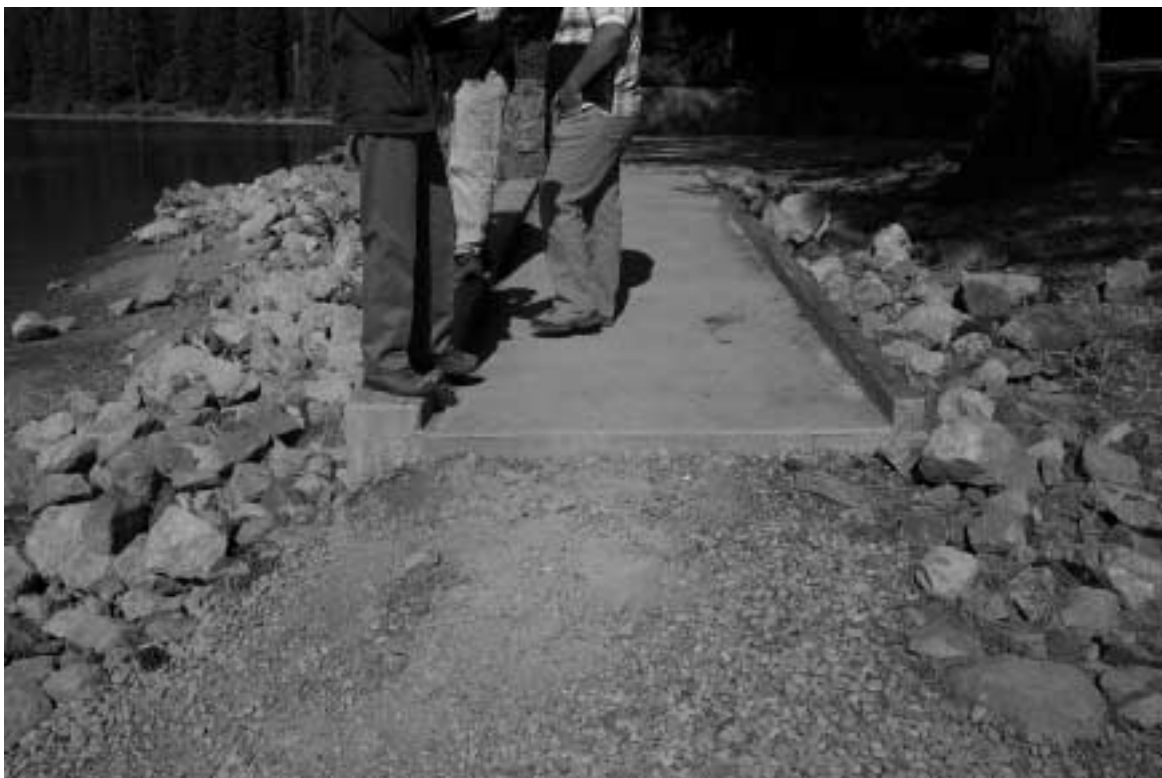
Photo 9. Lip and gravel at end of new accessible ramp at the Canyon Dam picnic area.
